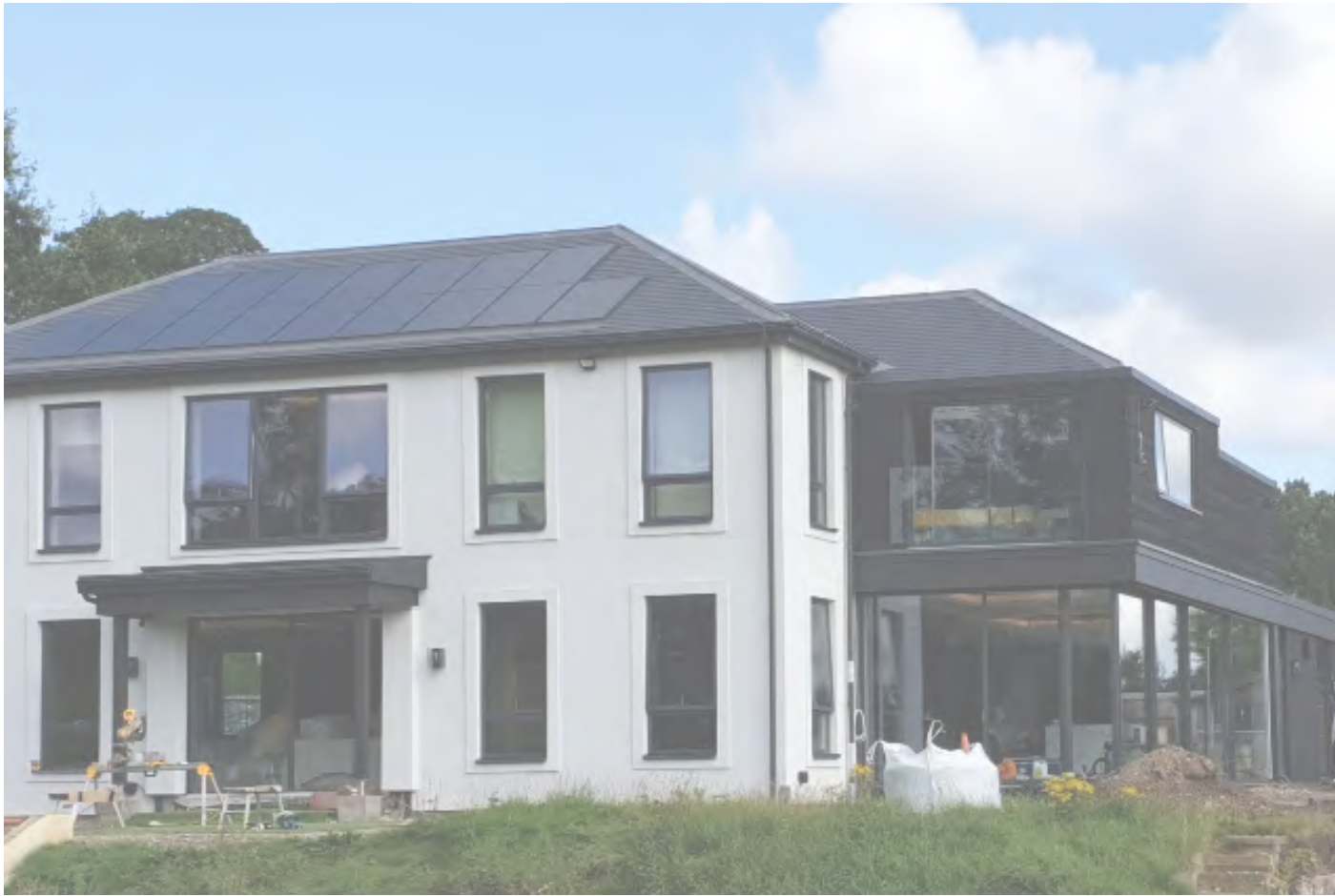
Top Project SOUTHBURN GRANGE
