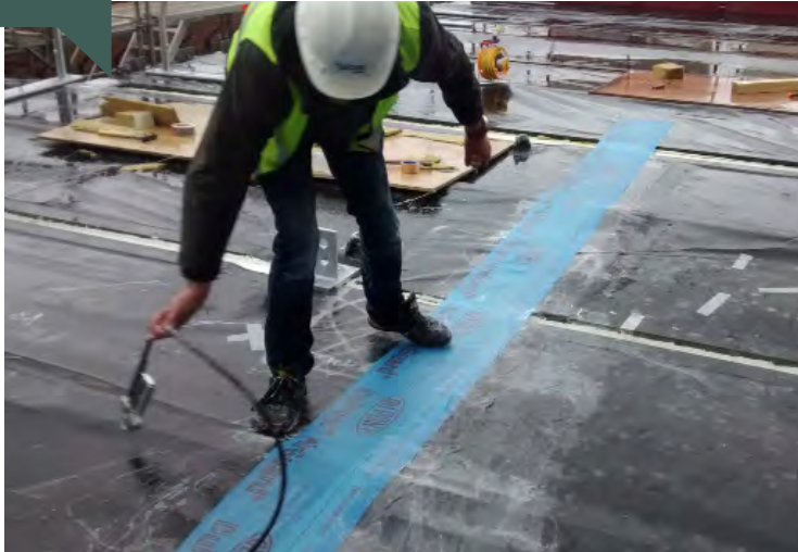
Joints between modules are sealed
