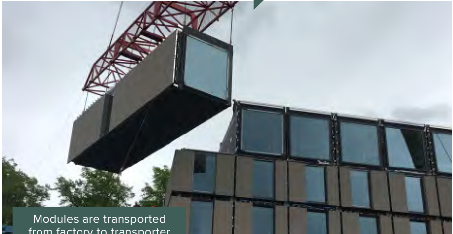
Modules are lifted into position by crane
